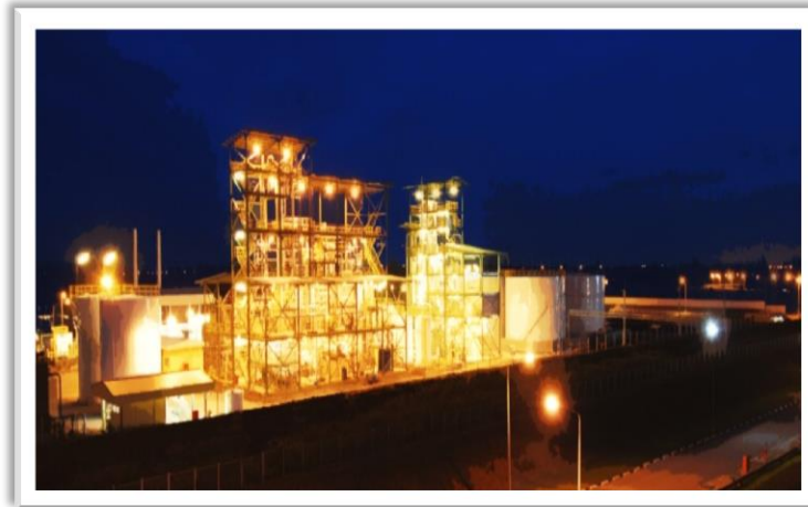
Mechanical Installation and Process Plant Construction for Energy and Petrochemical Industry
