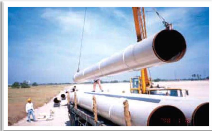
Pipeline Construction for Energy and Petrochemical Industry
