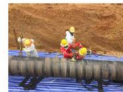
Figure 3. Prior to removal, the operation site is cleaned and every hole is provided the coating surface is wetted that will be removed in an upcoming pattern to avoid overloading of the steel.
