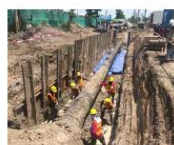
Figure 2. After excavation, the trencher was used to excavate the ground under the pipe to install the induction system. The trencher is a large machine that cuts through the soil, creating a narrow trench. The pipe is visible above the trench, and the trencher is positioned next to it.
