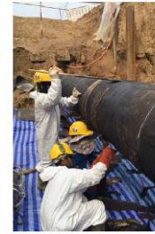
Figure 5. By moving the induction head over the pipe coating, the surface is heated to 140 – 160°C inside the coating is easily scraped off by using scrapers.
